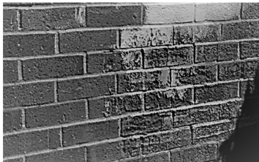
Effects of sandblasting on brick surfaces.
